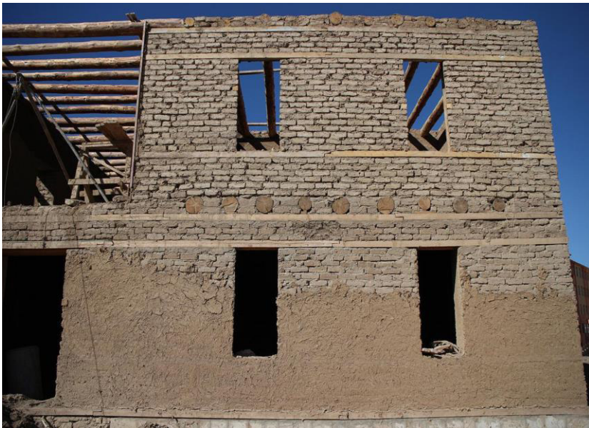
Figure 3 - Adobe house with anti-seismic presides
